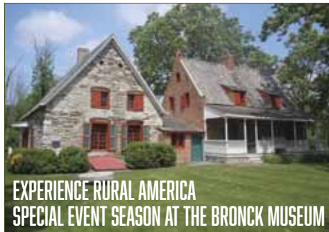
Visitors to Bronck Museum participate in guided tours of National Historic Landmark structures that reflect over three hundred and fifty years of architectural history.
